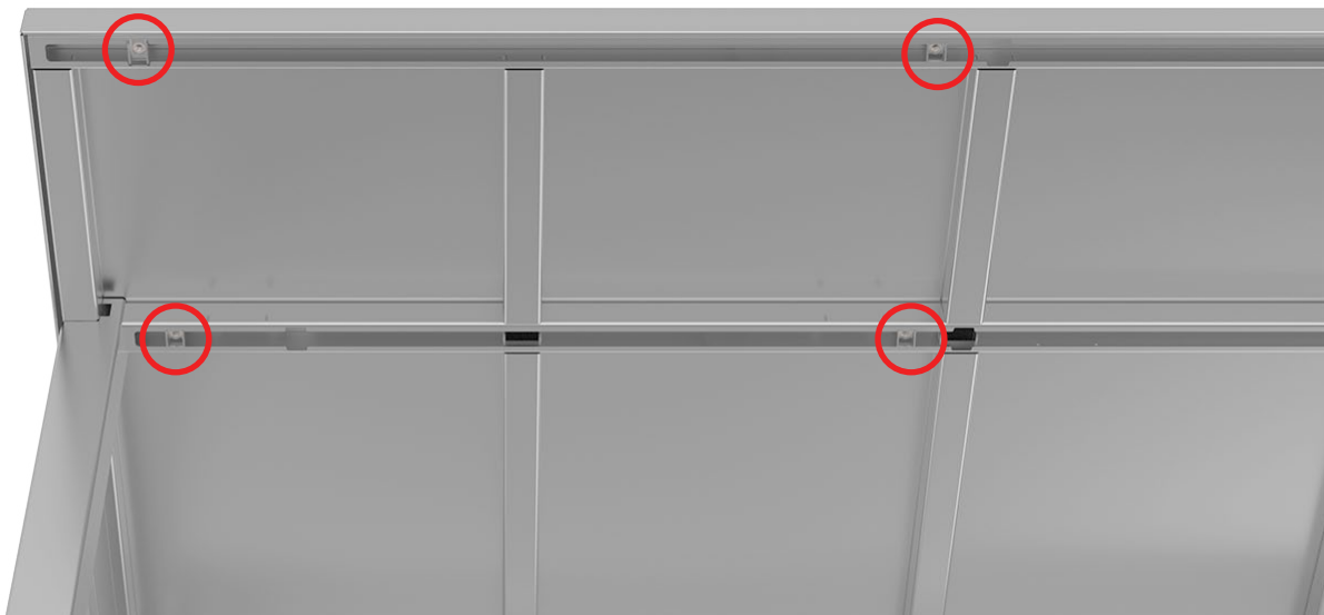
View from underneath
